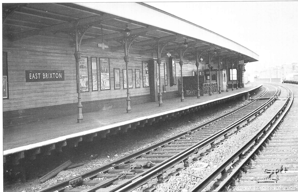
Top The LBSC side of Peckham Rye in its original form but after removal of the up fast track. In 1962 the original platforms were demolished and replaced by an island platform.
