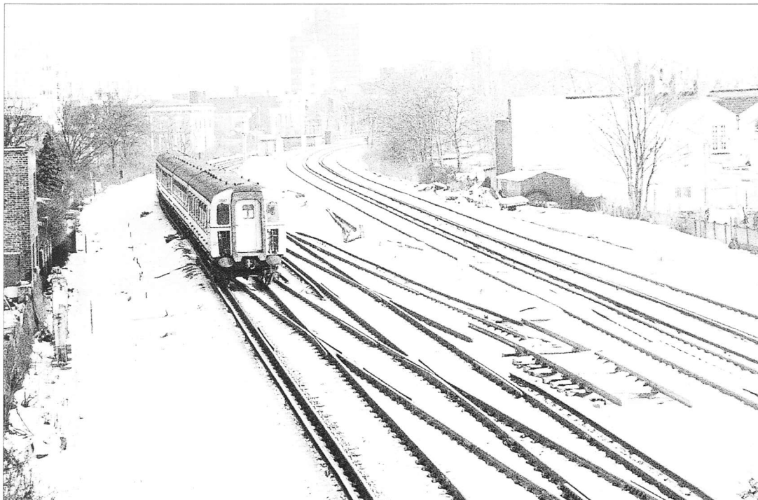
Looking towards Brixton on 14th February 1991. A down train for Bromley South and beyond passes a new connection being put in between the LCD lines to the left and the LBSC ones to the right. A.C. Mott
